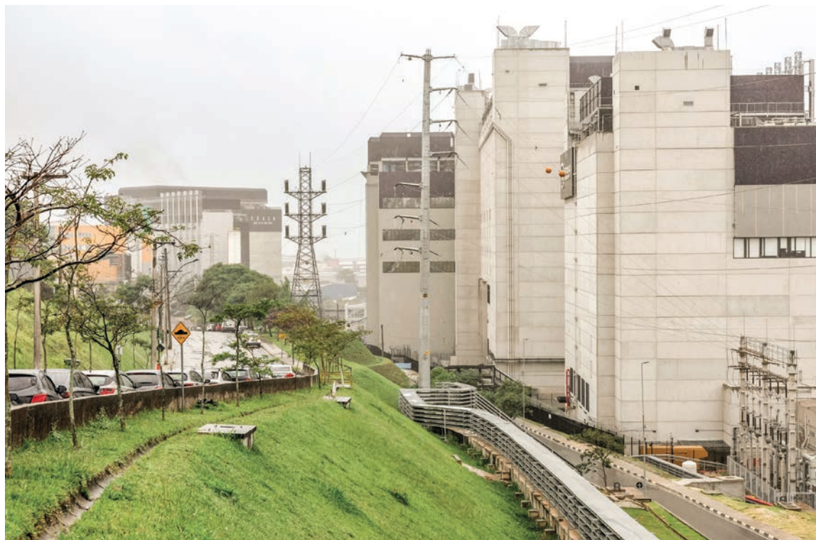
The Scala Data Centers Tamboré Campus in Barueri, Brazil, is one of the the largest and most advanced data center complexes in Latin America.
